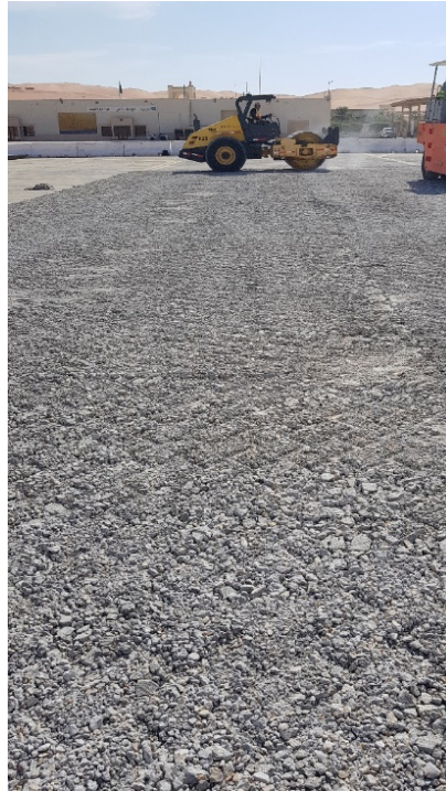
Figure 21. Roller compacted rubblized pavement.
