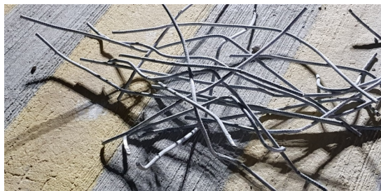
Figure 19. Reinforcement bars removed from pavement.
