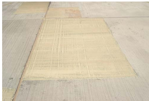
Figure 4. Concrete patch repaired (large size).
