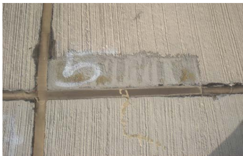
Figure 5. Concrete patch repaired (smaller size) with deformed joint sealant.
