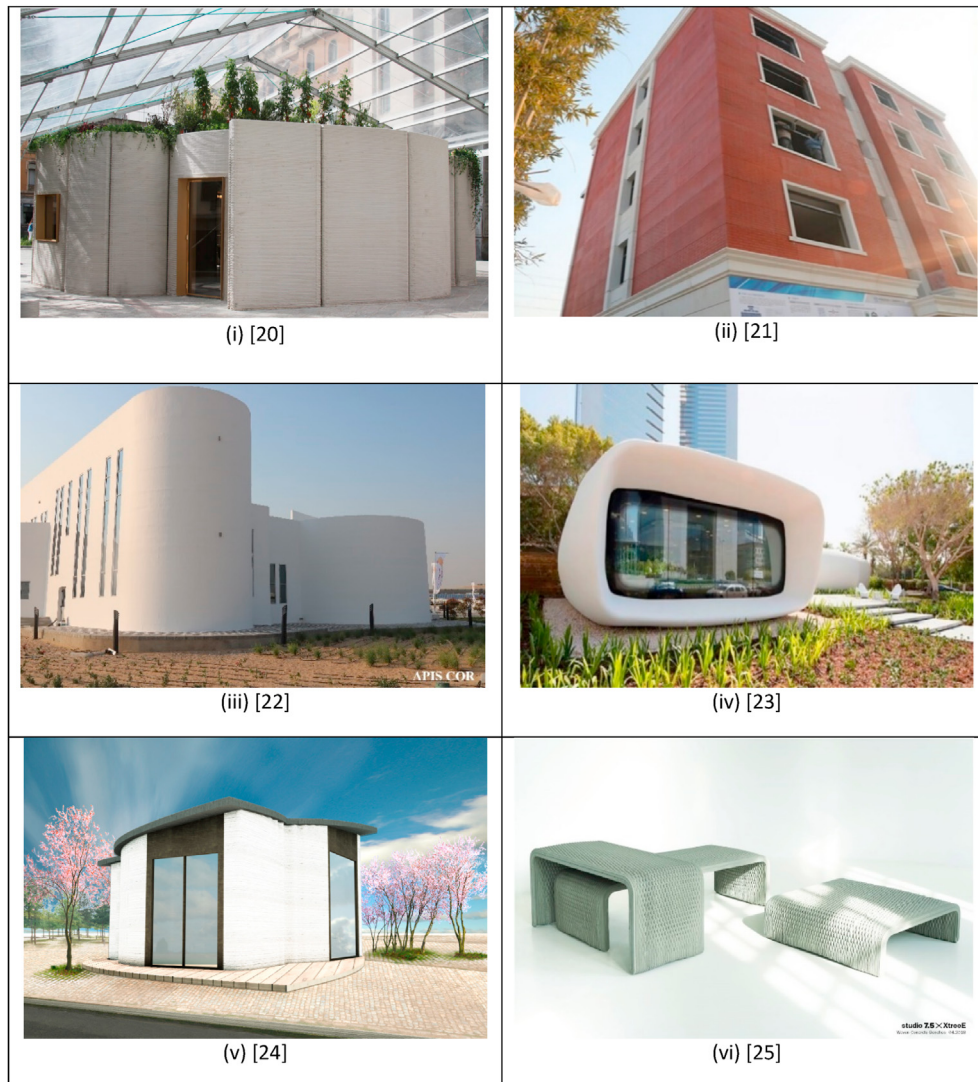
Fig. 1. Few real-world examples of 3D printing technology for concrete construction exist, from (Al Rashid et al., 2020): (i) 3D Housing 05, Milan (ARUP), (ii) 3D-Printed Multi-Story Apartment, Winsun (World's First 3D-Printed Apartment Complex), (iii) Double-Story Administrative Building in Dubai (Dubai Project - Apis Cor), (iv) First 3D-Printed Office in Dubai (World's First 3D-Printed Office Building Unveiled in Dubai), (v) Europe's First 3D-Printed Building (The BOD) (BOD2), (vi) Woven Concrete Benches (XtreeE)
